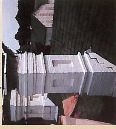
FIGURE 4: Pouring two separate flues for the furnace and fireplace.
