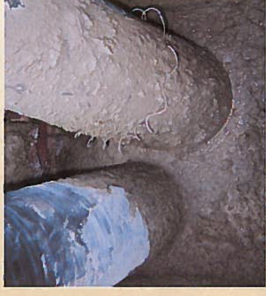
FIGURE 4: Pouring two separate flues for the furnace and fireplace.
